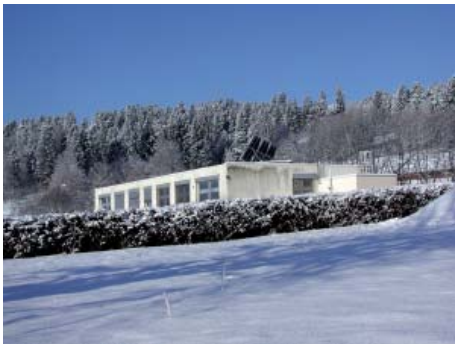
The Switch Craft Plant, 1100m above sea level
